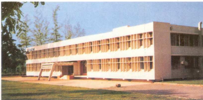
Manufacturing and Research & Development Centre, Navi Mumbai
